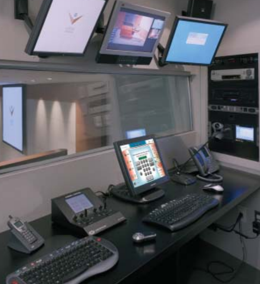
Crestron's e-Control and RoomView products give operators control over resources and allows the campus' AV operations to be run from a single control room.
